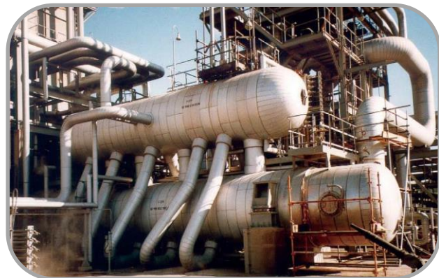
(up) Innovative Process Boiler design (down) Conventional Process Boiler design
